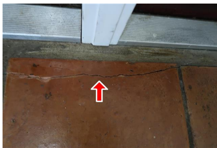
7.0 Item 1 (Picture) Front door
