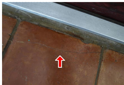
7.0 Item 2 (Picture) Front door
