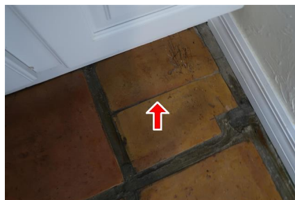
7.0 Item 8 (Picture) Kitchen
