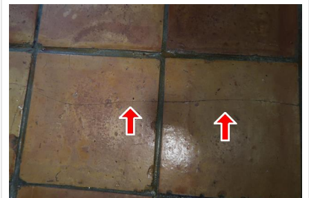
7.0 Item 6 (Picture) Shared bedrooms hallway
